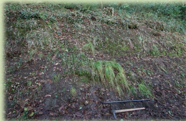
The site after clearance work with the plants visible in the centre of shot
